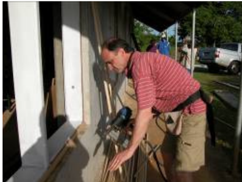
Nailing our fabricated quad onto the window frames.
