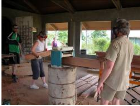
Libb and Jack machining timber for the windows.
