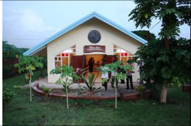
The front of the completed Chapel at dusk.
